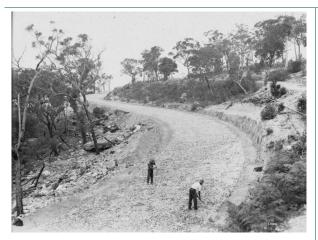
Figure 37. Photograph from 1928 taken by Main Roads Board, depicting highway labourers constructing the road foundation north of the study area, between Gosford and Mooney Mooney. Source: Western Sydney Records Centre, NRS-4481-3-[7/16010]-St13000
