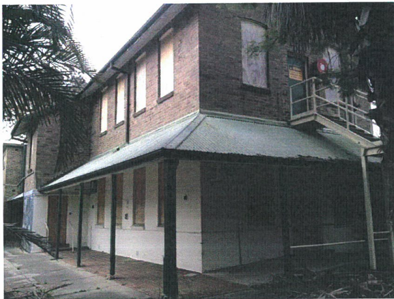
Western corner of Denby showing verandah, Image: Urbis, 2014
